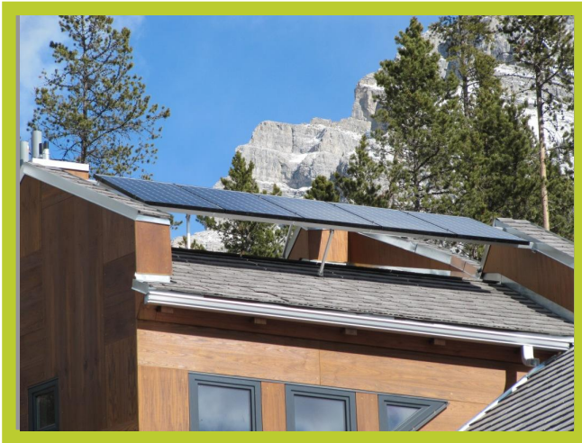
A KCP Energy solar electric photovoltaic install
